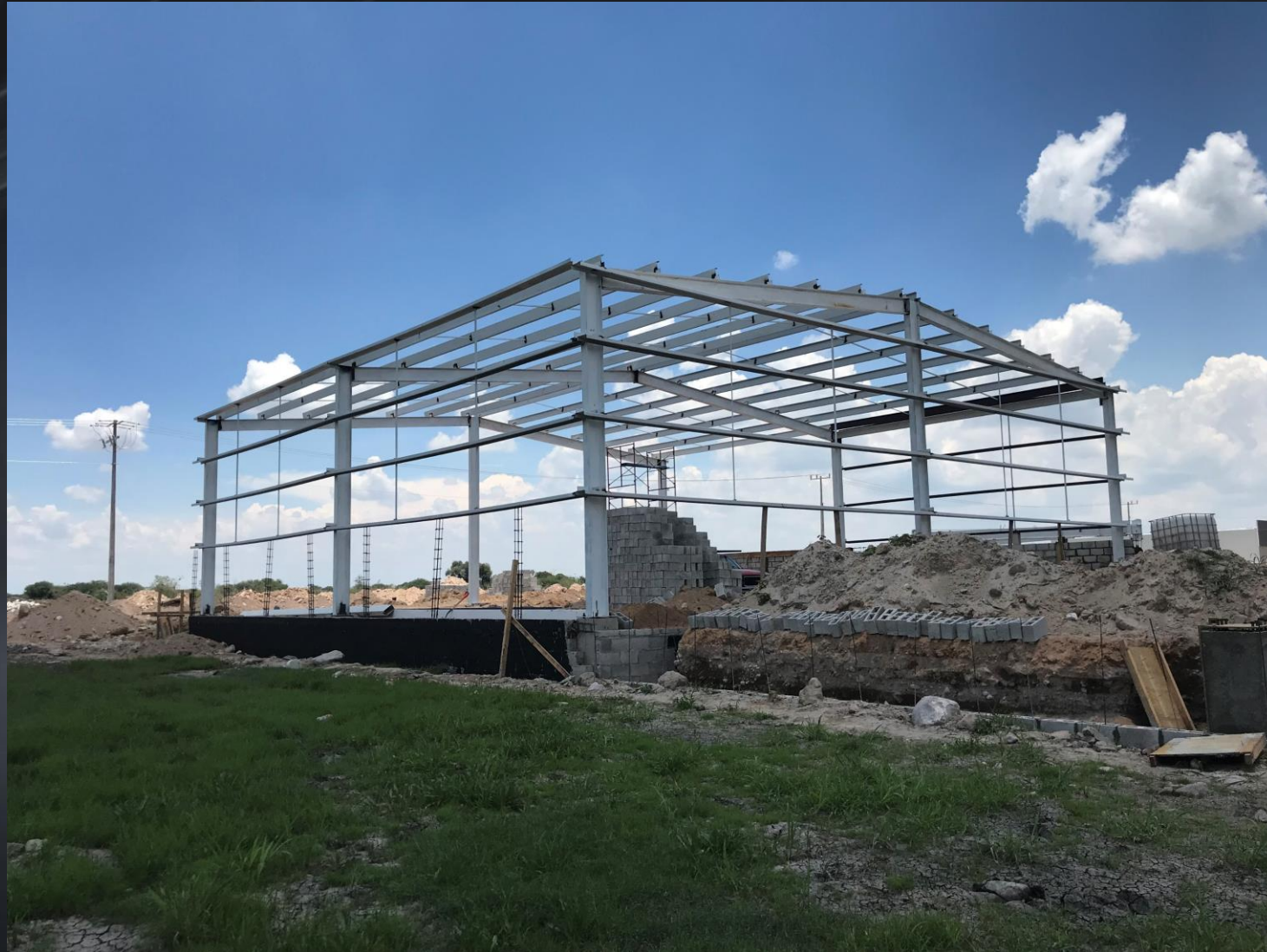
Nave industrial, ACRYLTEK S.A. de C.V.
